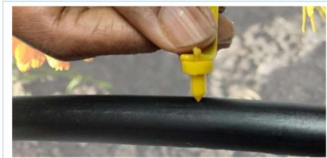
6. Make a punch in 16mm Main Line to insert 4mm feeder connection per plant
